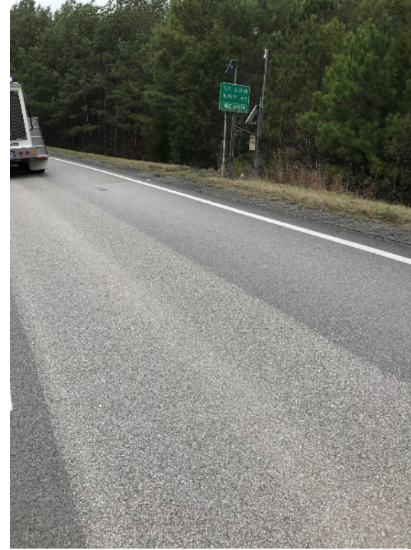
Shot blasted surface
