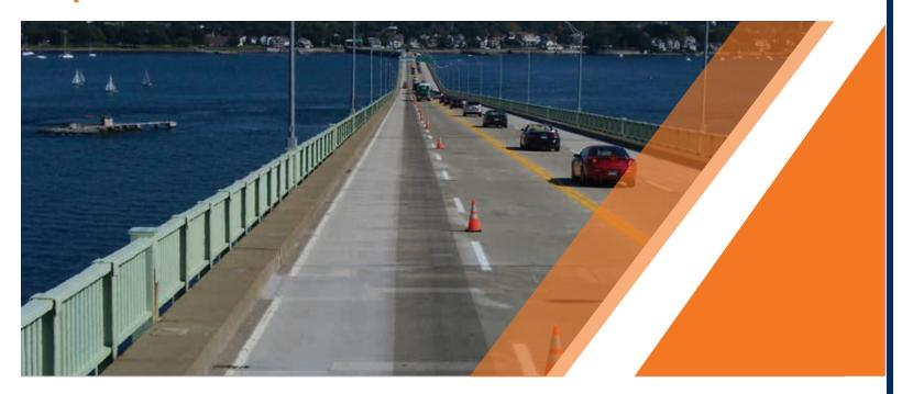
Elevated roadways present a unique challenge because the surface is susceptible to freezing. Without adding material, Skidabrader increases the micro and macro texture. This provides drainage and friction simultaneously without increasing the dead weight load limits and with minimal traffic disruption.
