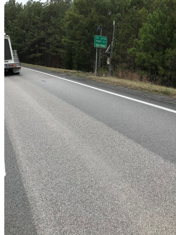
Shot blasted surface
