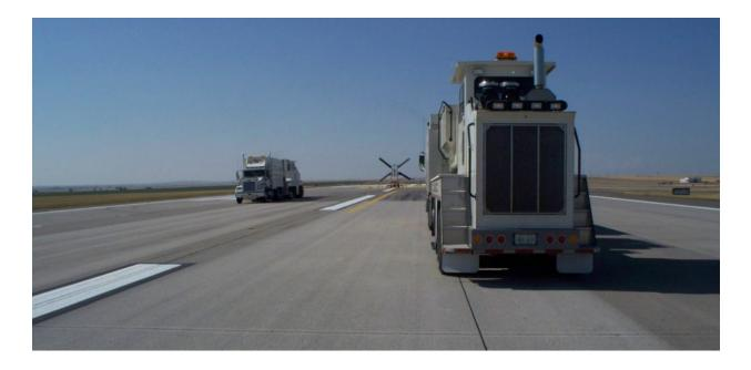
Waterblasting works similar to shotblasting but uses high pressure water instead of steel media. It is generally not as aggressive to the pavement surface as the mechanical texturing process and mainly removes rubber with little additional improvement of macrotexture. With the chemical cleaning method, chemicals are applied to the pavement and then washed off with lower pressure water. The chemicals breakdown the rubber without changing the pavement surface.
