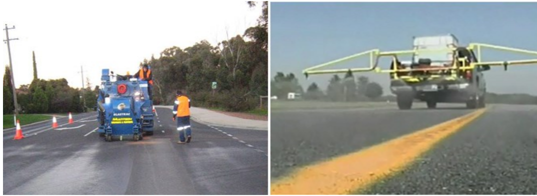
1 2 Figure 1. DOS -Treated Pavement: Shotblasting (Left), Densifier Application (Right) 3
